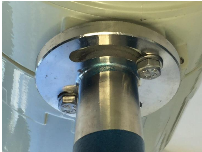
Connection Between Flow Converter and Flow Sensor To Be Sealed
