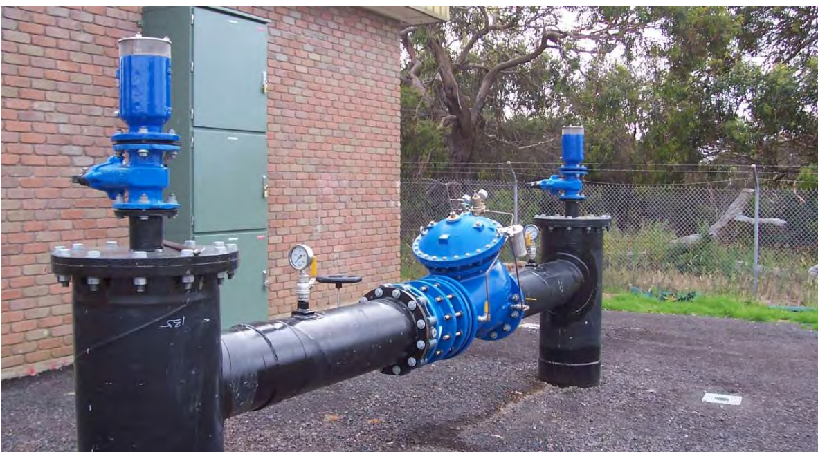
720 series-pressure reducing valve
