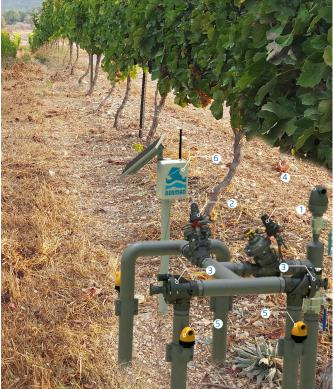
[1] BERMAD Model IR-120-DC-XZ reduces the supply pressure to preset pressure, protecting the system
