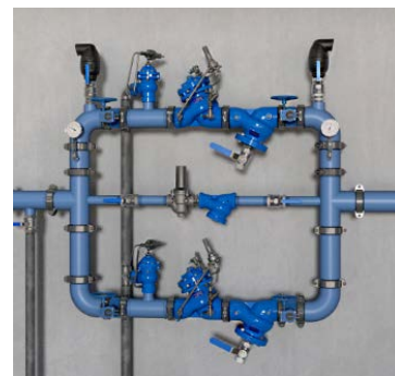
Picture 4.8 – On Floor pressure reducing station
