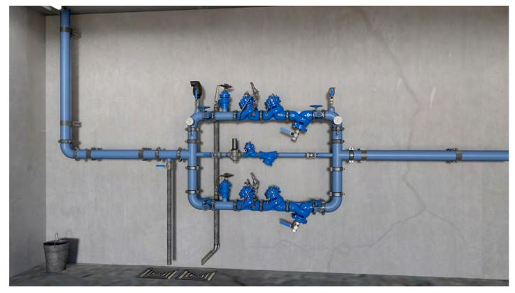
Two-Stage Pressure Reducing Station, featuring BERMAD BC-720-PD-P valves to reduce the incoming pressure by a fixed ratio and share the load with the BERMAD BC-720-P PRV, a redundant, parallel branch to minimize the possibility of total water shut-off and a low
